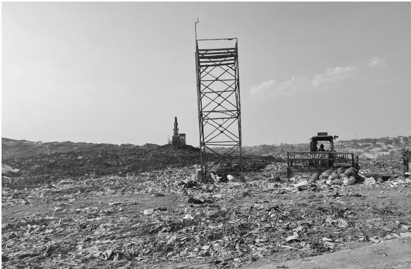
Fig. 15: Equipment Chunga landfill, Lusaka, October 2022 (own image)
