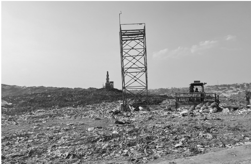
Fig. 15: Equipment Chunga landfill, Lusaka, October 2022 (own image)
