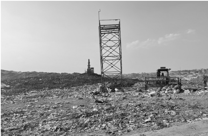
Fig. 15: Equipment Chunga landfill, Lusaka, October 2022 (own image)
